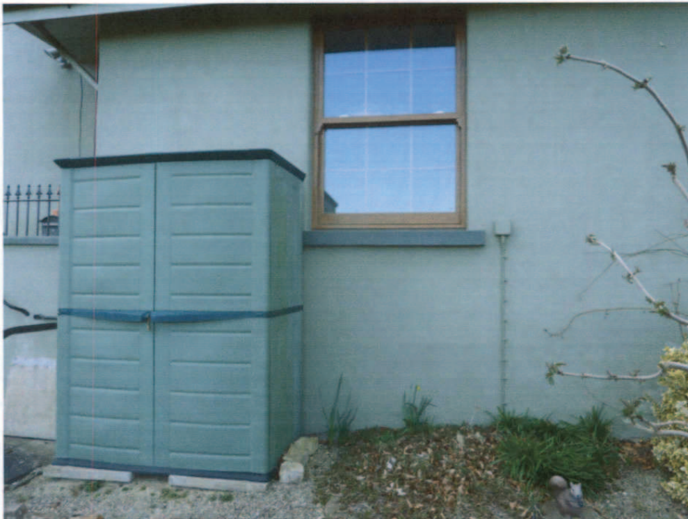
Proposed site of ASHP (replacing existing green shed)
